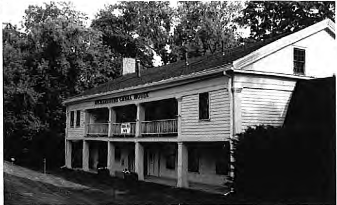
The Richardson Canal House complex provides a nice model for a design palette for the Old Erie Canal Sub-Area on Monroe Avenue
