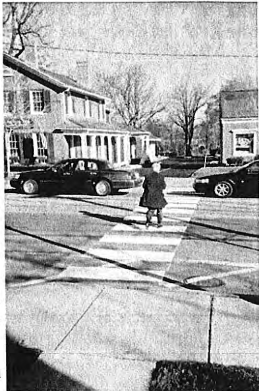
As an alternative to traditionally striped crosswalks this example shows large painted bands or “crossing bars”.
